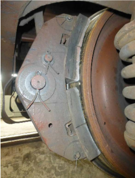
Melted brake block
